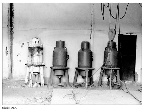
Figure 3: Seed Irradiators Used in the Former Soviet Union
